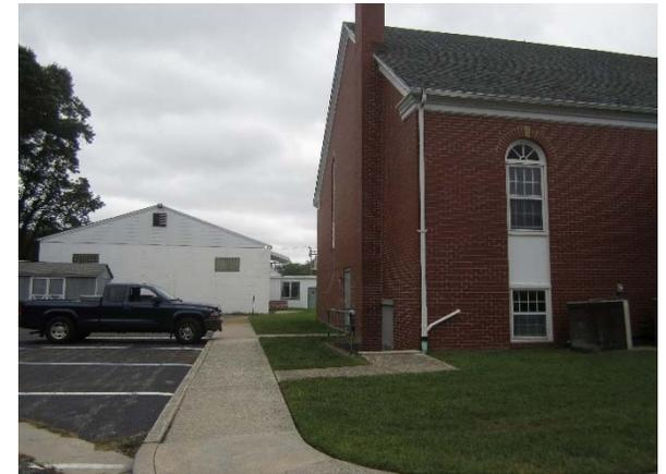
Installing a rain garden adjacent to the north side of the church can capture, treat, and infiltrate roof runoff. A preliminary soil assessment suggests that the soils have suitable drainage characteristics for green infrastructure.
